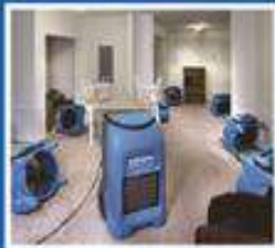
Structural Drying
